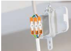
Lighting connection in suspended ceilings
