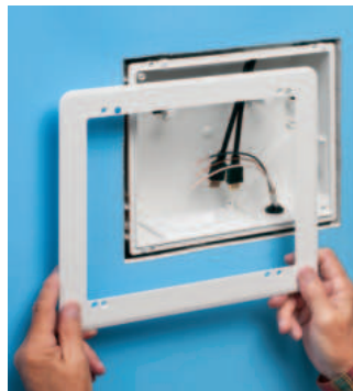
Attach trim plate with screws provided.
